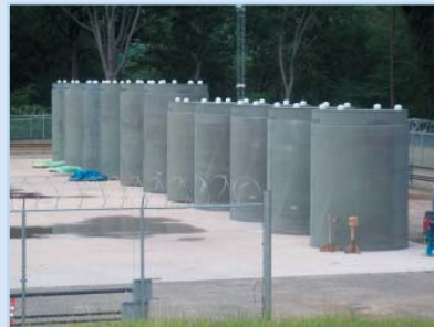
The smaller casks will hold the fuel components from the Unit 1 spent fuel pool.
